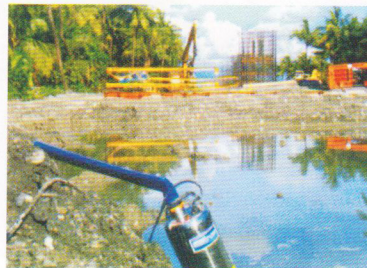
●Dewatering for civil engineering.
