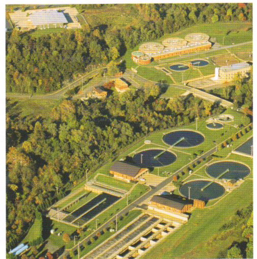
● Multi-drainage waste water treatment plant.
