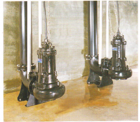
● TOS Guide rail system installation
